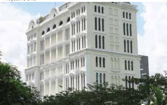
Le centre commercial Paragon Shopping center, Vietnam
